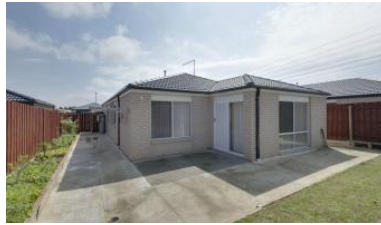
7 Tiarne Crescent, Hampton Park
