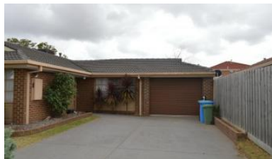
34 Leopold Crescent, Hampton Park
